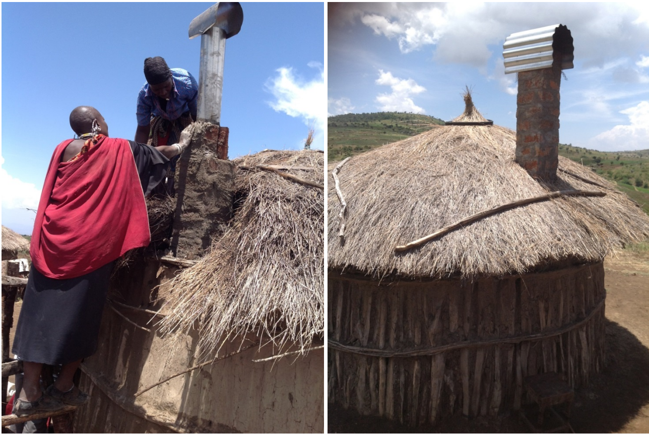
Figure 7. Women in Monduli installing the Maasai stove (left); installed chimney (right). Photo courtesy AWF.
