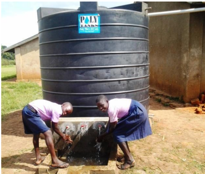
Pupils at Karongo Primary School in Uganda washing their hands at the newly installed water tank in their school. Photo Credit: JGI
